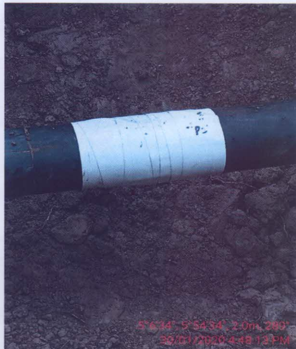
INCIDENT POINT AFTER REPAIR
